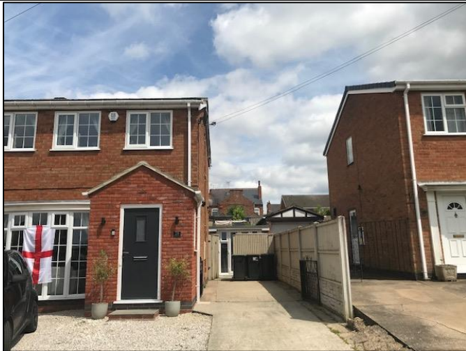
Photograph showing existing front elevation of the dwelling and where the proposed two storey side extension would be located.
